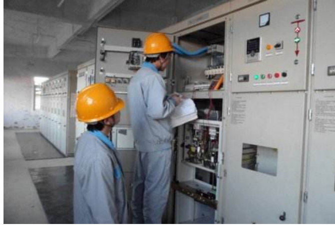
Figure 2 Commissioning of high voltage mechanical and electrical equipment
